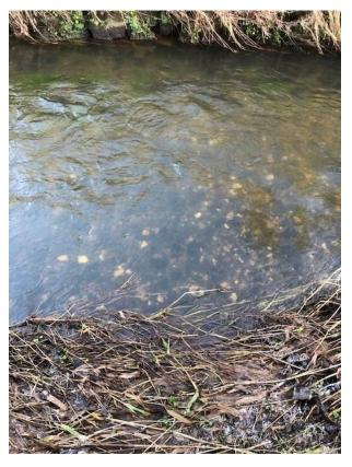
The length of the bank erosion is 18 meters, to repair this bank I would use willow posts and woody brash, which is plentiful on site due to the storm damaged caused by the recent storm.
